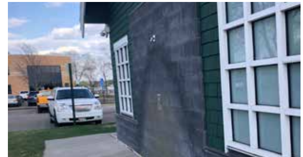
Existing showers hidden behind the building.
