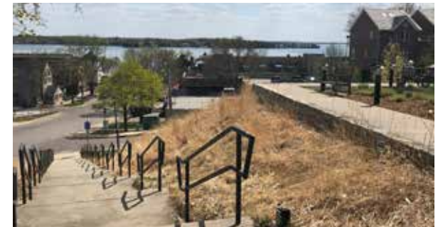
Existing Stairway leading to Lake Street
