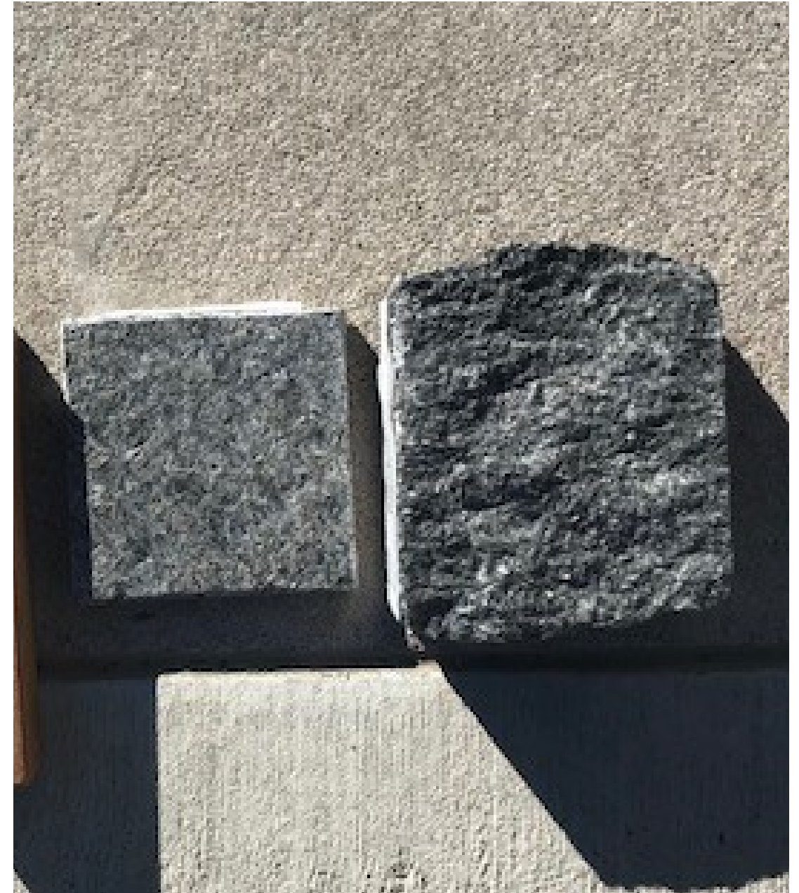
Granite base meeting concrete
