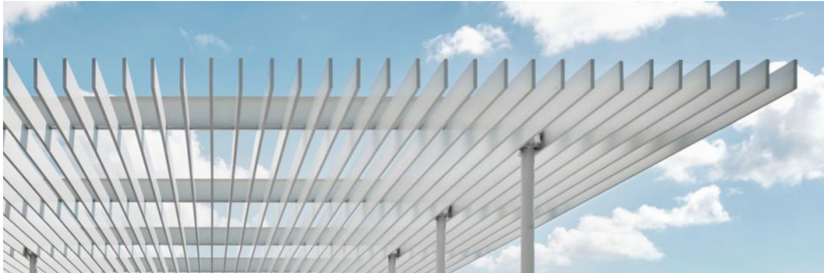
Vertical white battens connect to the shade canopy structure
