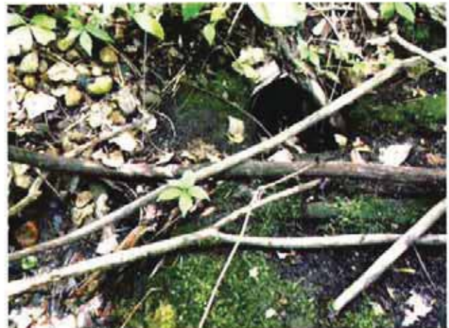
Wetland 1 inlet pipe, viewing east
