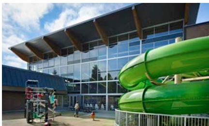
LYNNWOOD RECREATION CENTER CITY OF LYNNWOOD, WA
