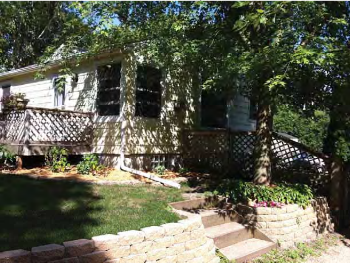
SW Corner of Existing Structure
