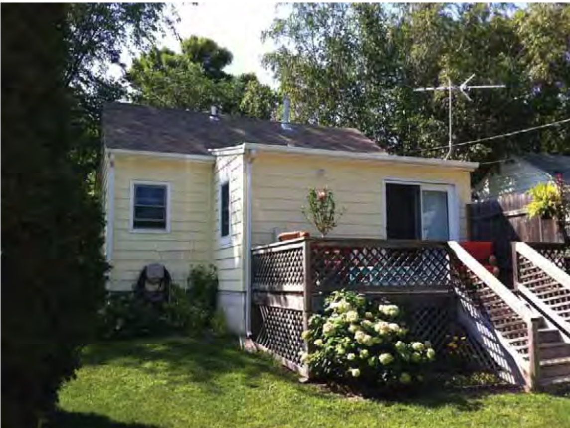
SE Corner of Existing Structure – Rear of Structure – Looking West
