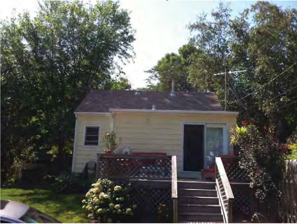
Rear Façade of Existing Structure – Looking West
