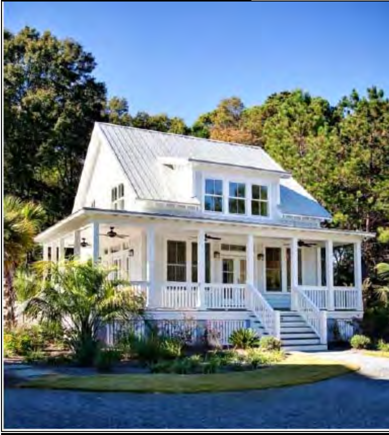
Image 1: Example of Roof Addition
