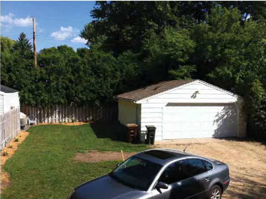
Existing Garage and Rear Yard – Looking East from Existing House
