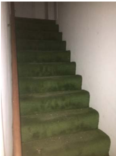
Fig. 1.45 Stairs to second level
