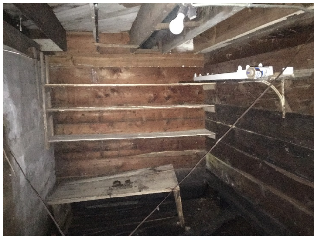
Fig. 1.31 Smaller storage room below 1943 addition
