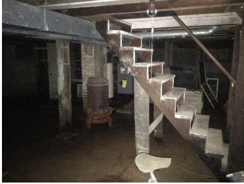
Fig. 1.64 Stair at basement level
