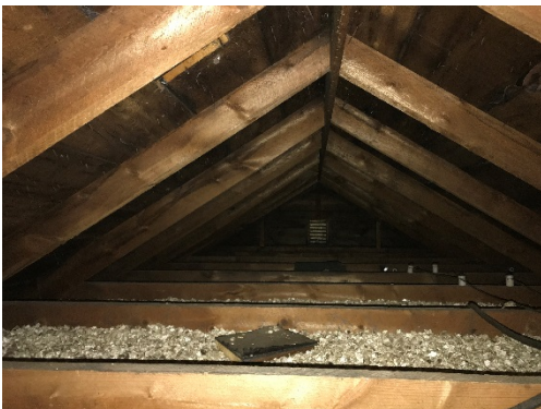
Fig. 1.25 Attic of original structure with vermiculite insulation
