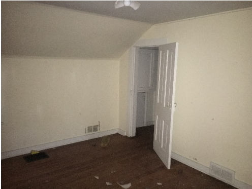
Fig. 1.60 Painted wood door at second level
