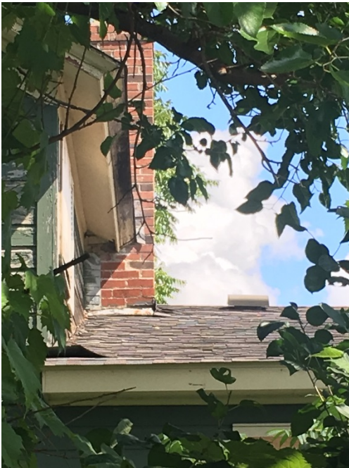
Fig. 1.24 Roof intersects with original southern façade
