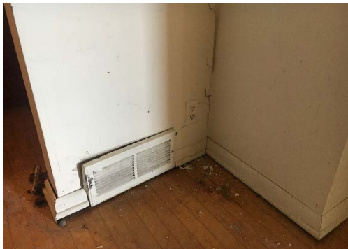
Fig. 1.67 Baseboard at living room near chimney
