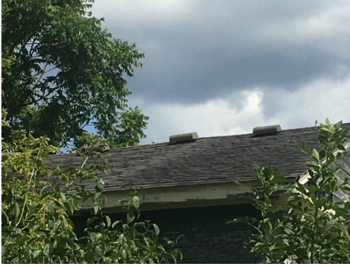
Fig. 1.23 Image of roof over addition looking east
