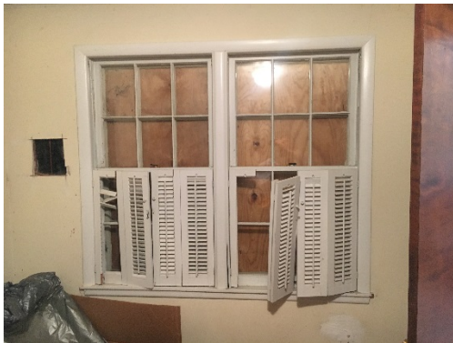
Fig. 1.18 Window at south addition – bedroom
