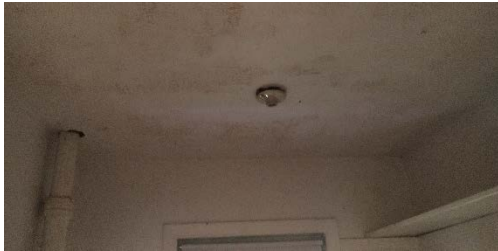
Fig. 1.52 Ceiling of Laundry Room
