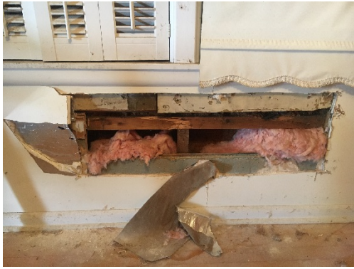
Fig. 1.20 Selective demolition below west kitchen window
