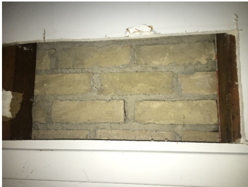
Fig. 1.27 Interior Chaska cream brick chimney at the closet demolition area showing struck joints
