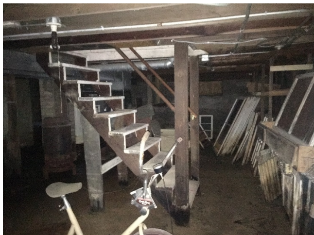
Fig. 1.30 Basement stairs below 1902 structure
