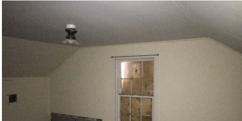
Fig. 1.50 Fiberboard wall and ceiling at second level
