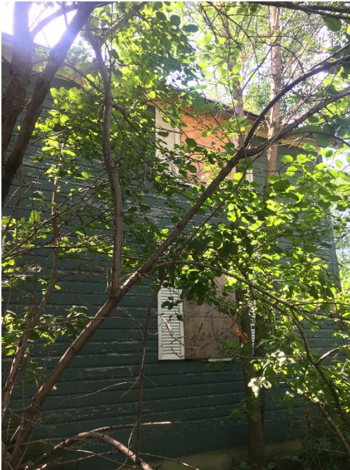
Fig. 1.1 Portion of north façade showing the original, two-story house
