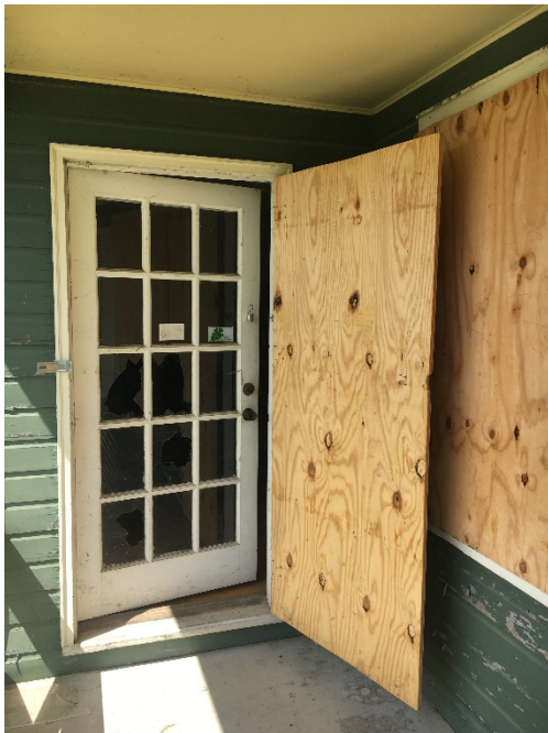
Fig. 1.15 South addition entrance at porch
