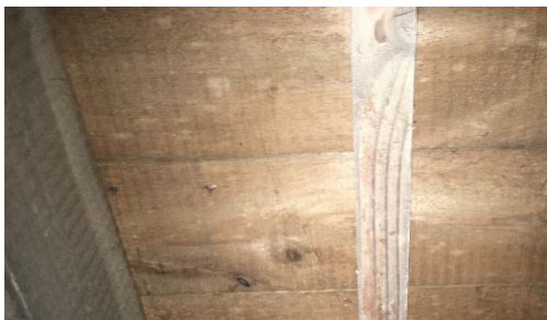
Fig. 1.58 Horizontal floor boards of original building as seen from basement
