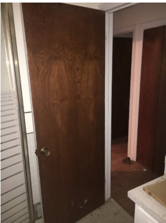
Fig. 1.62 Stained/painted wood doors on first level
