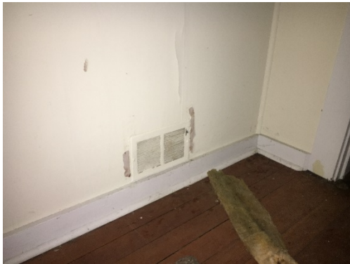
Fig. 1.66 Baseboard in second level bedrooms
