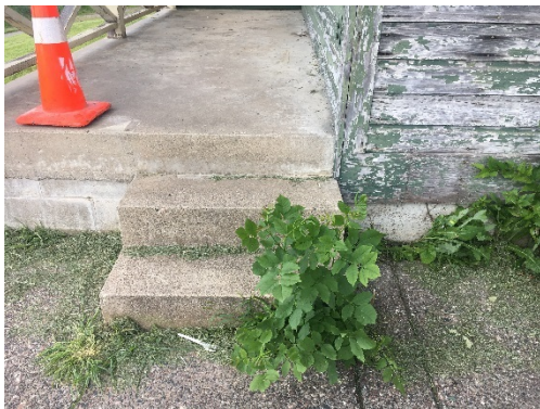
Fig. 1.11 Poured concrete foundation intersection with CMU block foundation on the east end at the 1960's addition
