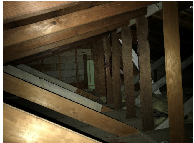
Fig. 1.44 Attic above additions
