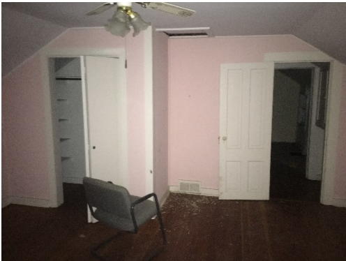
Fig. 1.61 Folding wood door at second level
