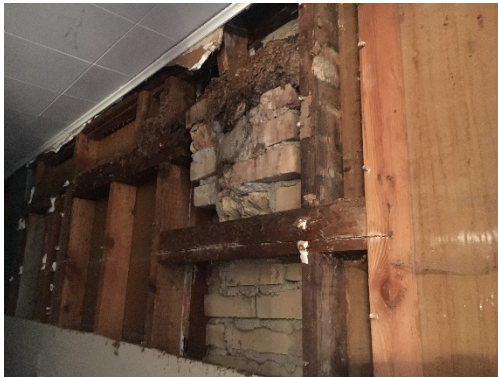
Fig. 1.21 Selective demolition at original south wall
