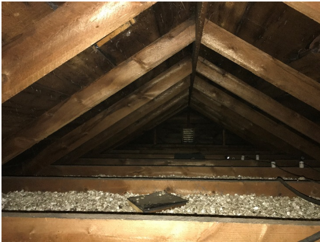
Fig. 1.43 Attic above bedrooms
