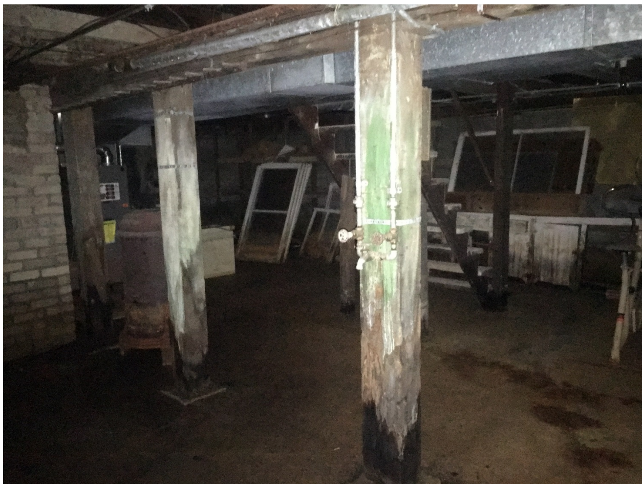
Fig. 1.32 Wood columns and beam in center of basement
