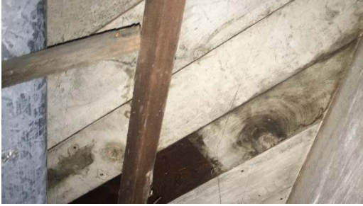
Fig. 1.59 Diagonal floor boards of addition as seen from basement
