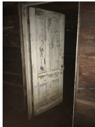
Fig. 1.63 Original painted solid wood door in basement may have been relocated
