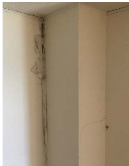
Fig. 1.53 (left) crack at second addition
