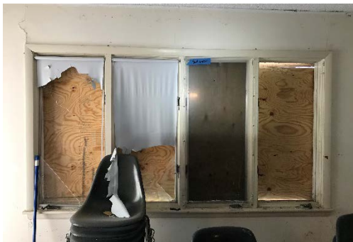
Fig. 1.19 Window at south addition – living room
