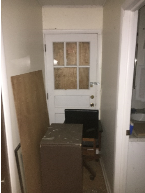
Fig. 1.14 East entrance original opening
