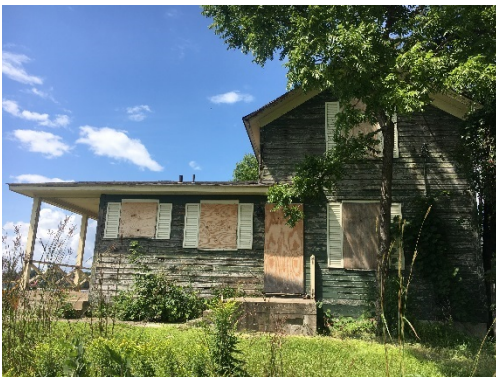
Fig. 1.2 East façade showing addition on left and original house on right
