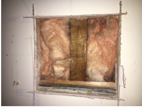
Fig. 1.46 Selective demolition on first level exterior wall
