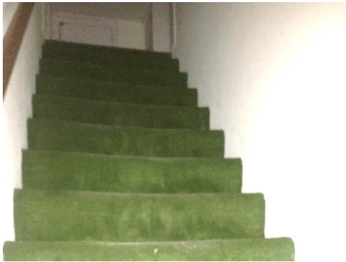
Fig. 1.65 Stair looking up to the second level landing from the first level entrance
