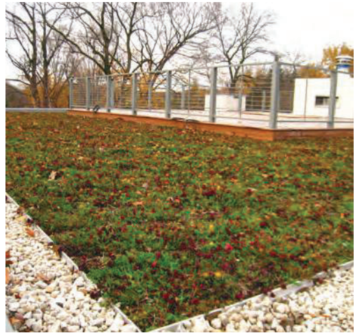
SEDUM EXTENSIVE ROOF
