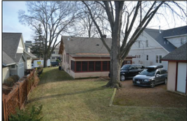
REAR OF 225 MANITOBA AVENUE SOUTH CITY OF WAYZATA, HENNEPIN COUNTY, MN
