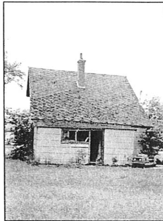
The front and side (left photograph) and back (right) of a section house of similar design in Henricks, Minnesota, in 1900. It has suffered a number of alterations since its construction in the late nineteenth or early twentieth century.
