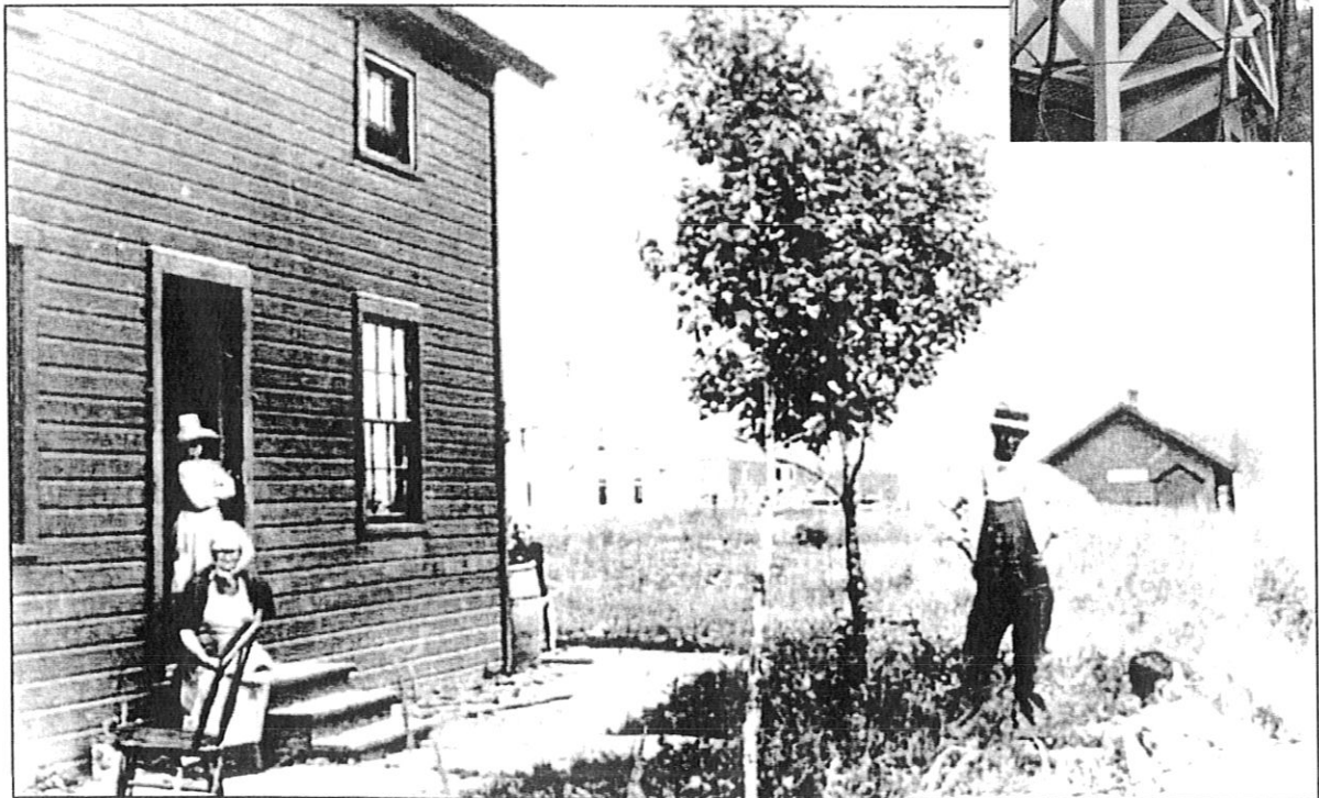
Askov section house (below), and detail of Wayzata section house (right). (Historic photograph from Minnesota Historical Society Collections)
