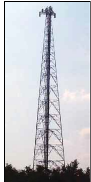
Typical Self Supporting Tower
