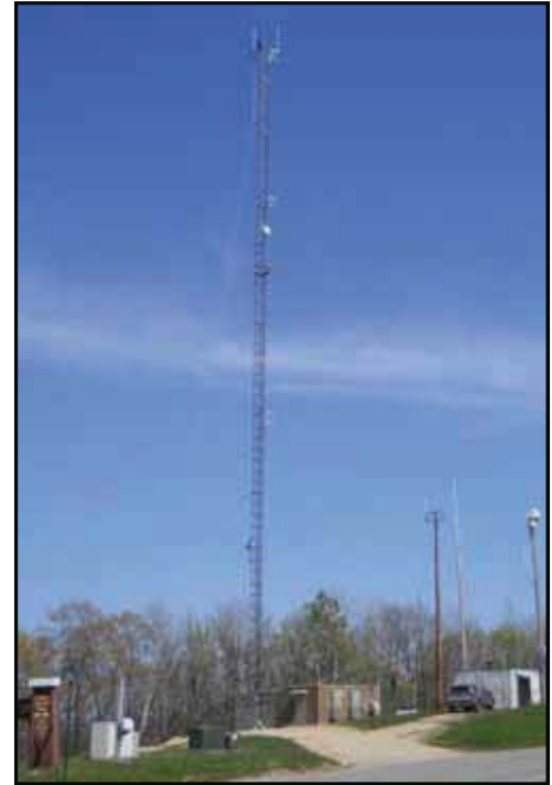
Typical Guyed Tower
