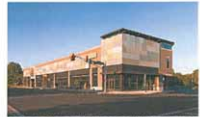
BROAD RIPPLE VILLAGE PARKING GARAGE
