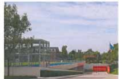
CHESAPEAKE ENERGY CENTRAL CAR PARK
