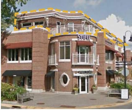
Fig. 3.35 Upper story stepback in a mixed-use building.
