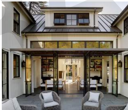
Fig. 3.31 A building recess provides a gracious entry to a restaurant
