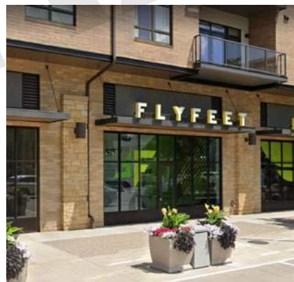
Fig. 3.43 Storefront with expansive glazing
