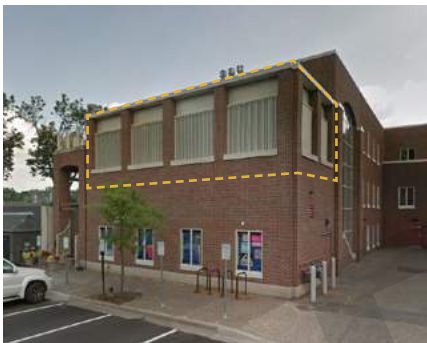
Fig. 3.51 Aerial view and street view of concealed rooftop equipment at the second floor / stepback level.
