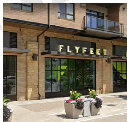
Fig. 3.43 Storefront with expansive glazing
