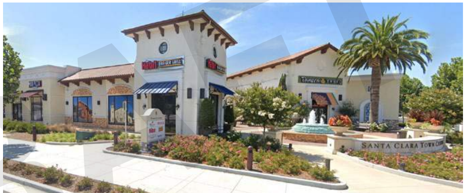
Fig. 2.6 Commercial centers with active frontages towards the street and corner open spaces.
