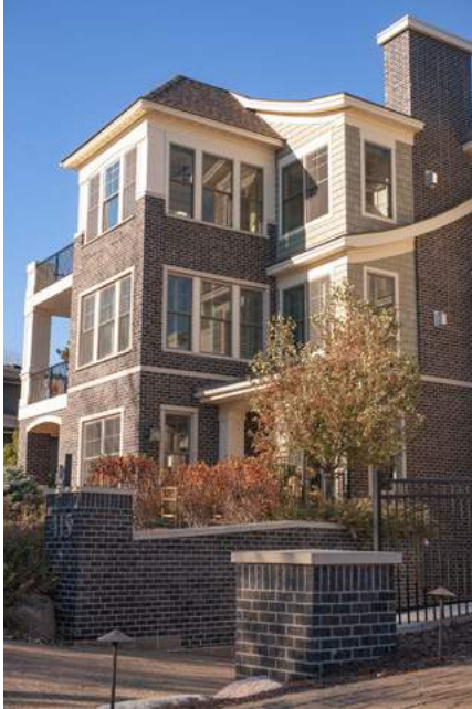
Fig. 3.61 Board siding material used on levels above masonry material on primary walls.
