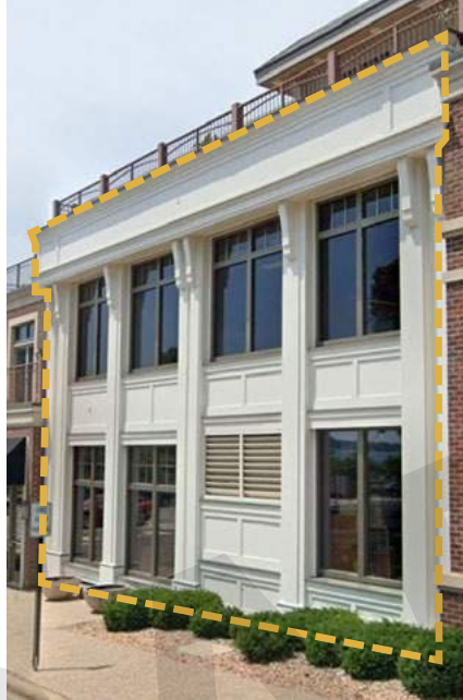
Fig. 3.62 One material and color unifies this two story element
