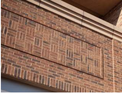
Fig. 3.6 Masonry trim and detailing provides fine-grain character and interest.
