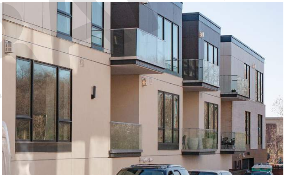
Fig. 3.64 This building demonstrates a simpler façade treatment at the rear driveway (bottom) than at façades facing public rights of way (top). Walls at private driveways, rear façades, and the interior of properties may provide muted materials and articulation.
