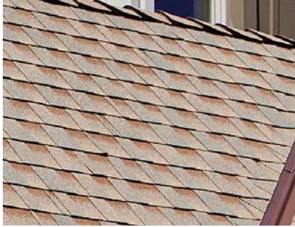
Fig. 3.14 Dimensional ('architectural') asphalt shingles provide more shadow than 3-tab
