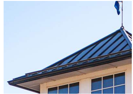
Fig. 3.16 Metal roofing in a neutral color complementing the building's color palette.
