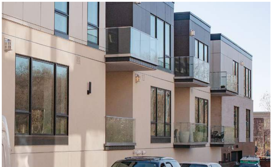
Fig. 3.62 This building demonstrates a simpler façade treatment at the rear driveway (bottom) than at façades facing public rights of way (top). Walls at private driveways, rear façades, and the interior of properties may provide muted materials and articulation.
