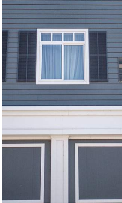
Fig. 3.3 Fiber cement lap siding with wood window trim, horizontal projecting trim, and wood pilaster are complementary Board Siding Materials
