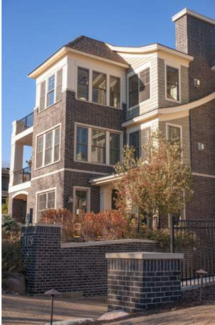
Fig. 3.59 Board siding material used on levels above masonry material on primary walls.
