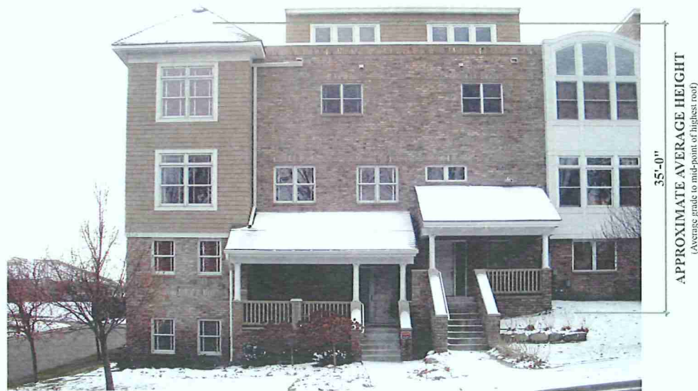
712 RICE STREET EXISTING STRUCTURE
