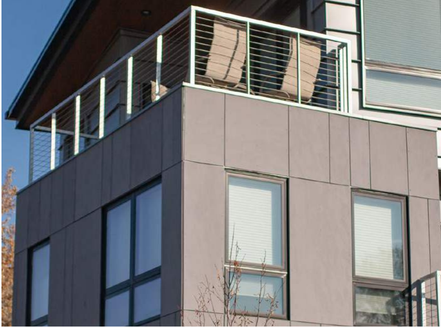
Fig. 3.12 Stucco joints relate to the proportions of this building mass.
