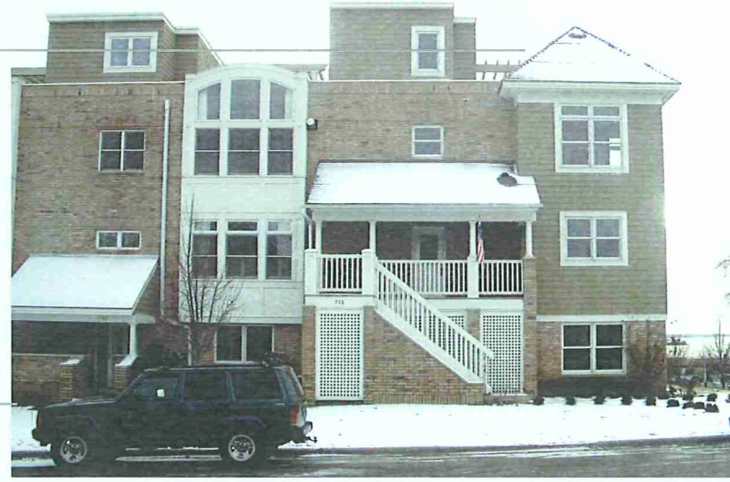
706 RICE STREET EXISTING STRUCTURE
