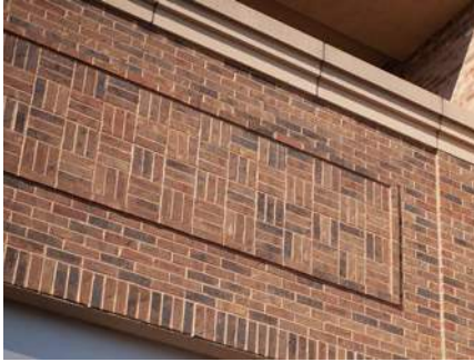
Fig. 3.7 Masonry trim and detailing provides fine-grain character and interest.
