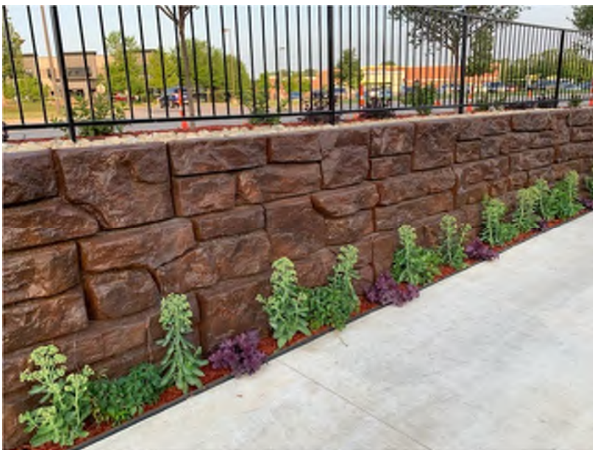
Figure 2: Stone textured retaining wall with accent railing, and plantings.
