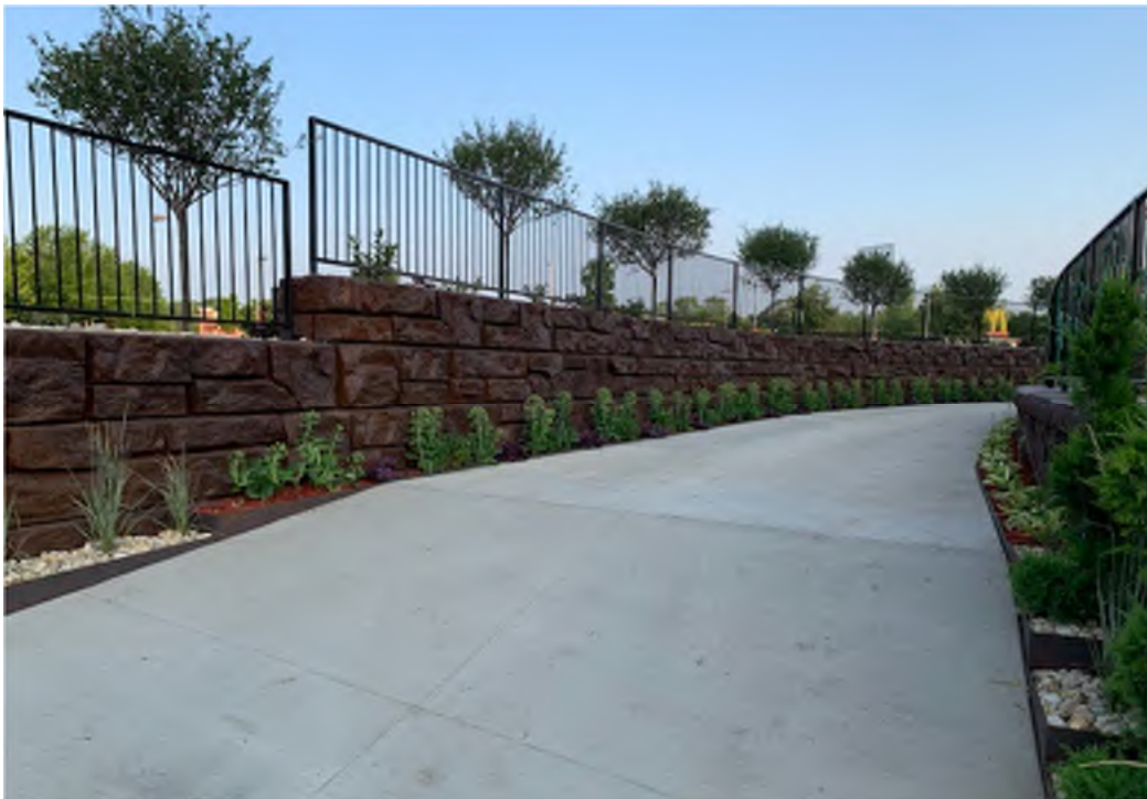
Figure 1: Service drive with retaining walls, plantings, and decorative railings.
