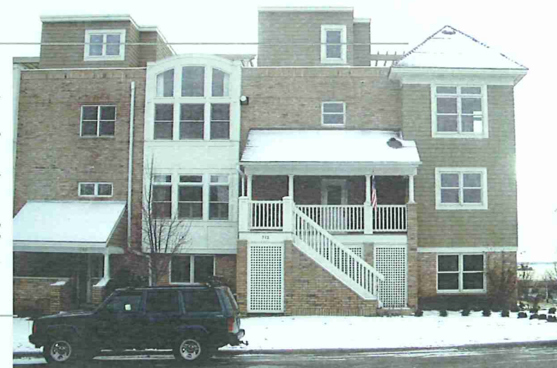
706 RICE STREET EXISTING STRUCTURE
