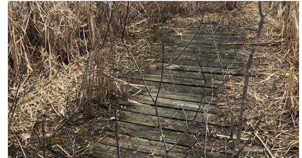
The old boardwalk remnants still exists.
