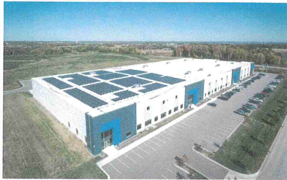
Flat Roof with Fully Ballasted Array (Compare to City Hall, Police/Fire, Library, and Rear of Muni Building)
