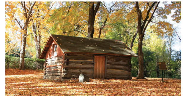
Existing historic Trapper's Cabin.
