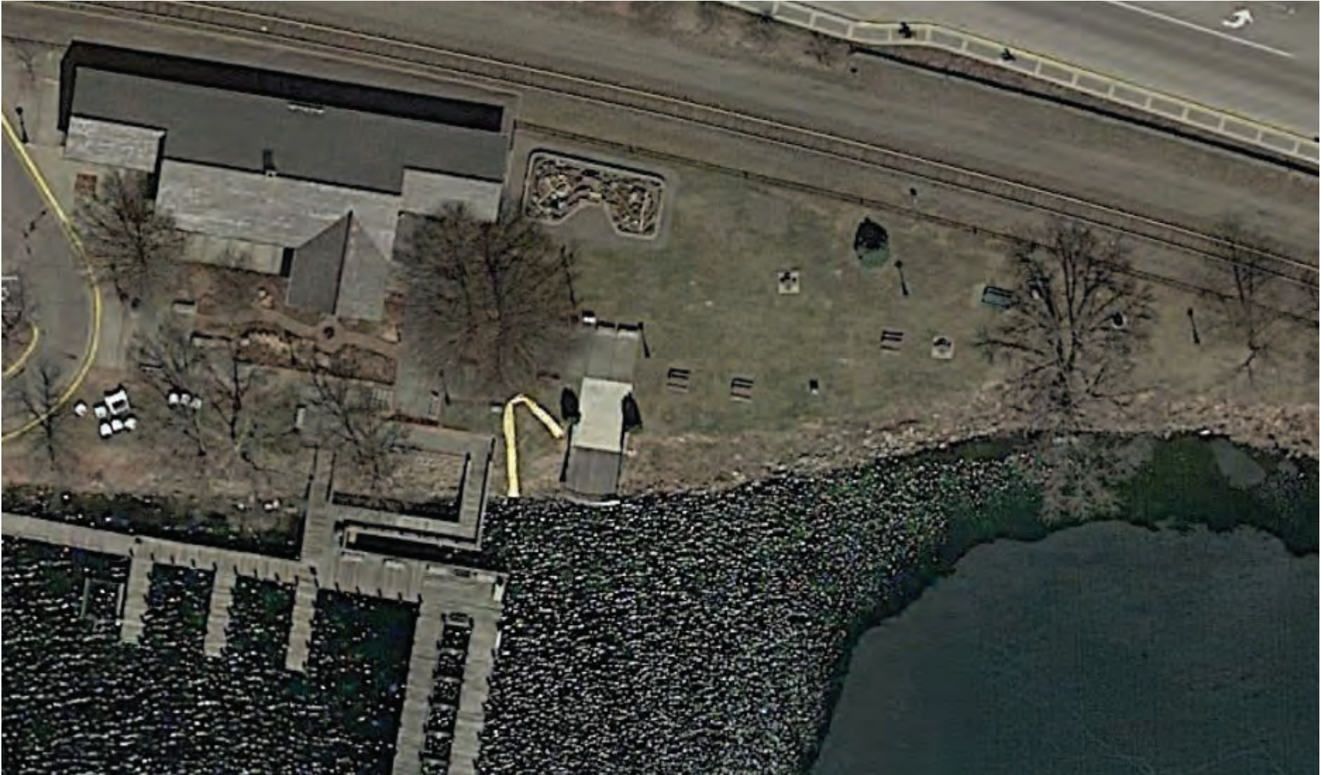
WAYZATA DEPOT PARK EXISTING CONDITIONS
