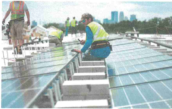
Flat Roof with Fully Ballasted Array (Compare to City Hall, Police/Fire, Library, and Rear of Muni Building)
