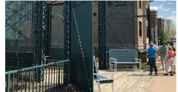
Existing entry gateway/sculpture.
