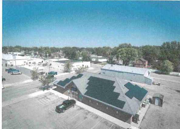
Pitched Roof with Asphalt Shingle (compare to Muni Building)
