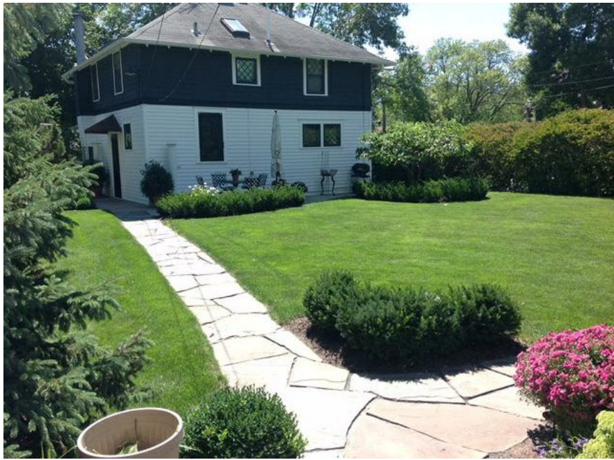
EXISTING NORTH FACADE
