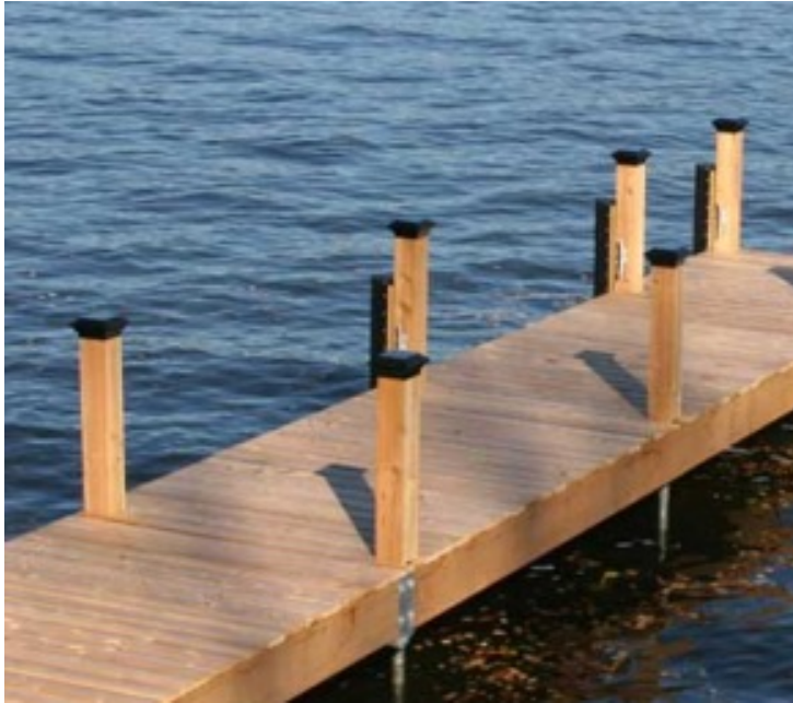
WOOD COVERED PILES
