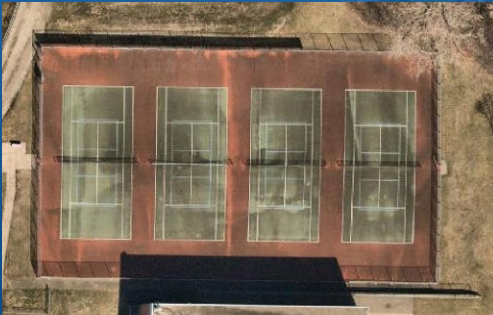
Wayzata Middle School – Reconstruct four tennis courts in existing footprint
