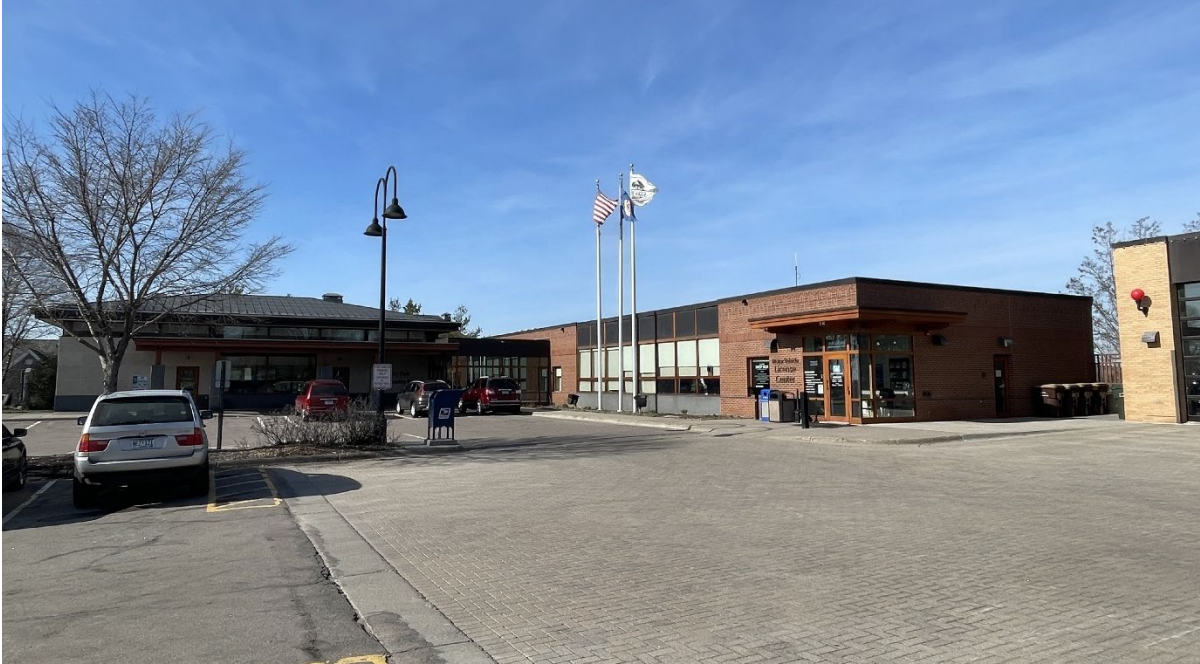
Image 2: City Hall from the main parking lot area.
