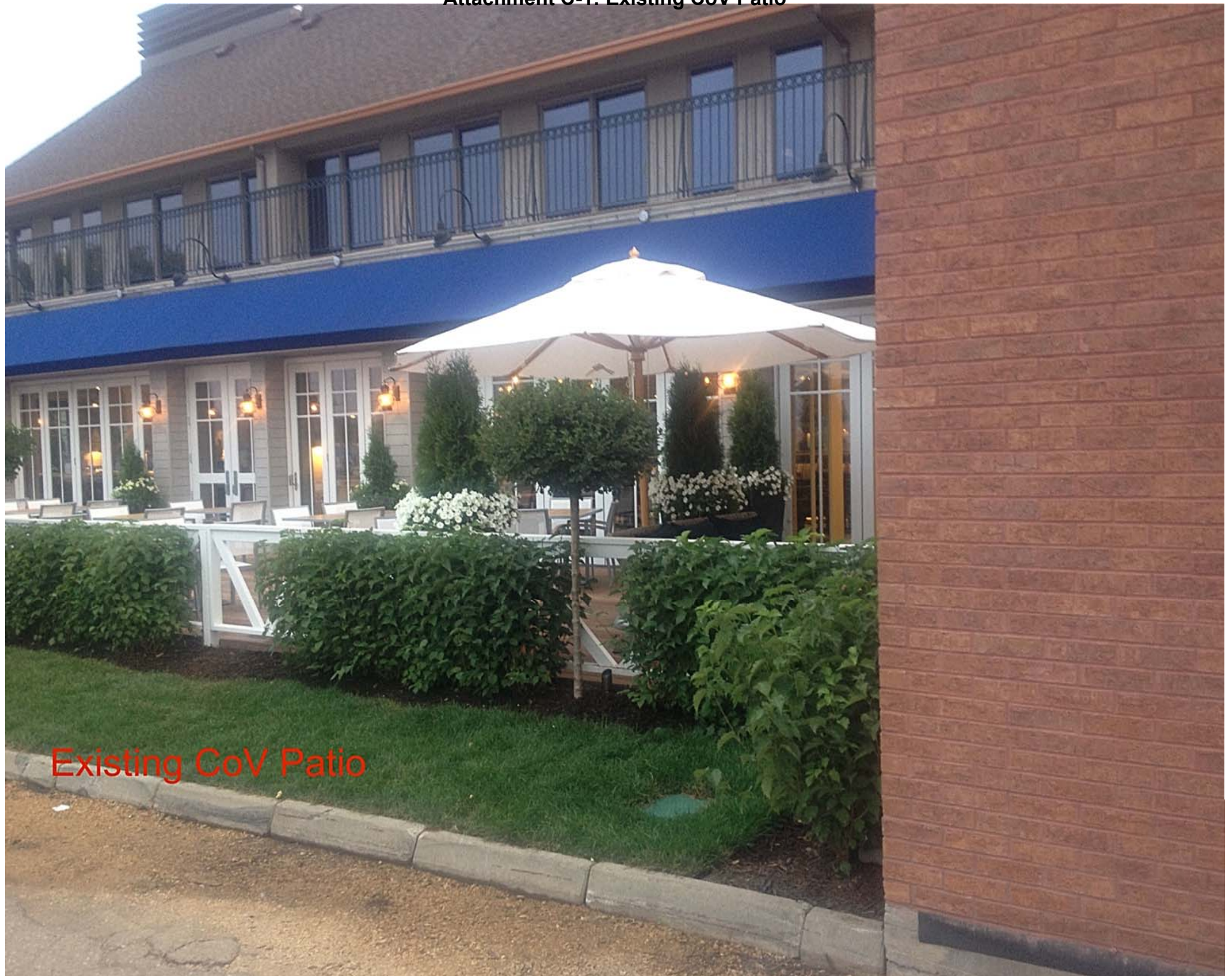
Attachment C-1: Existing CoV Patio
