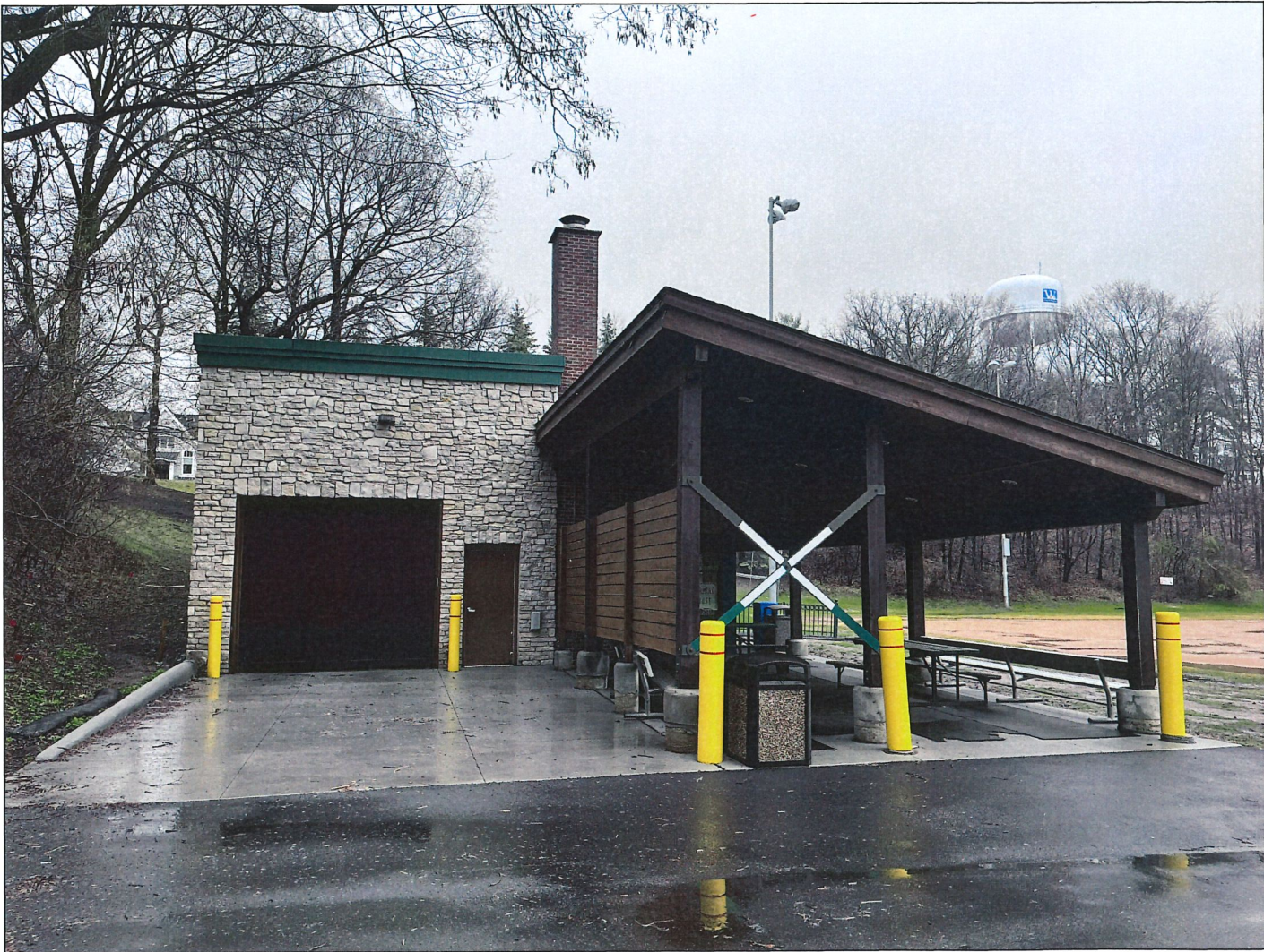
Photos of Existing Warming House Building
