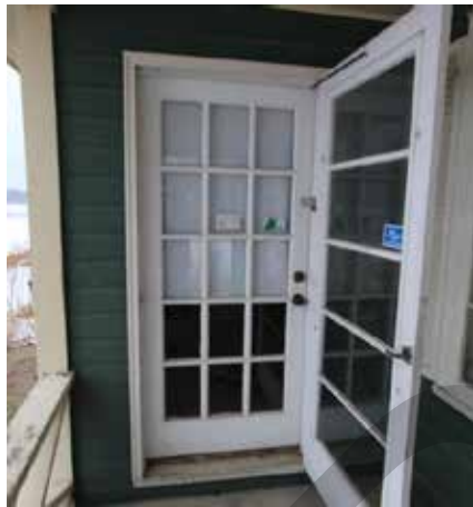
Figure 1.17 South addition entrance
