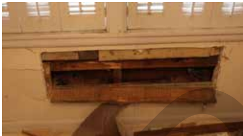
Figure 1.22 Selective demolition below west kitchen window
