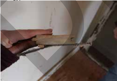
Figure 1.51 Cross section of tongue and groove wallboard with felt and wallpaper attached.
