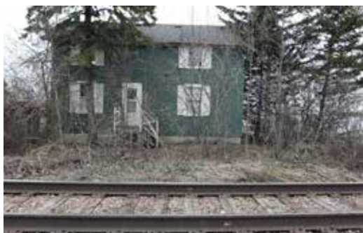
Figure 1.1 North façade of house as seen from railroad tracks (original entrance).
