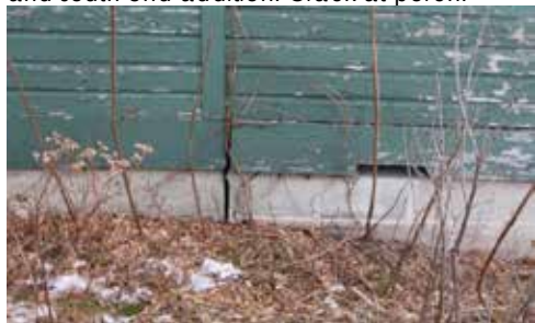
Figure 1.11 Poured concrete foundation meets CMU block foundation on the west end at the 1960's addition.
