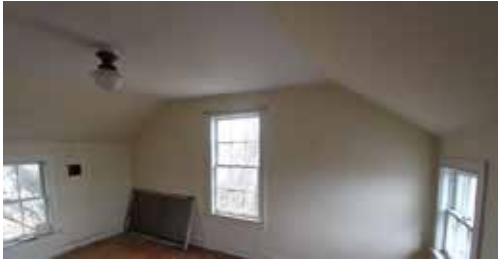
Figure 1.53 Sample of fiberboard wall and ceiling at second level.
