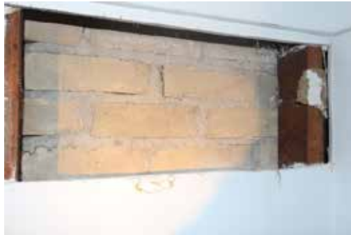
Figure 1.29 Interior Chaska cream brick chimney at the closet demolition area showing struck joints.
