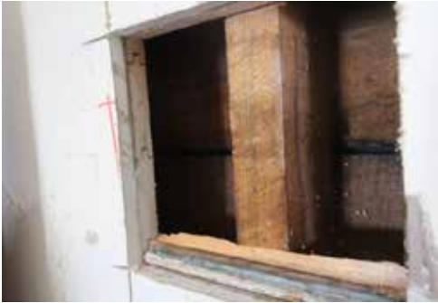
Figure 1.48 Selective Demolition on first level exterior wall.
