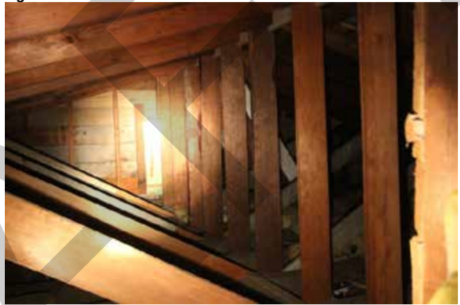
Figure 1.46 Attic above additions
