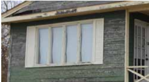
Figure 1.21 Window at south addition living room
