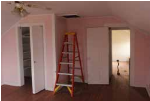
Figure 1.64 Folding wood door second level
