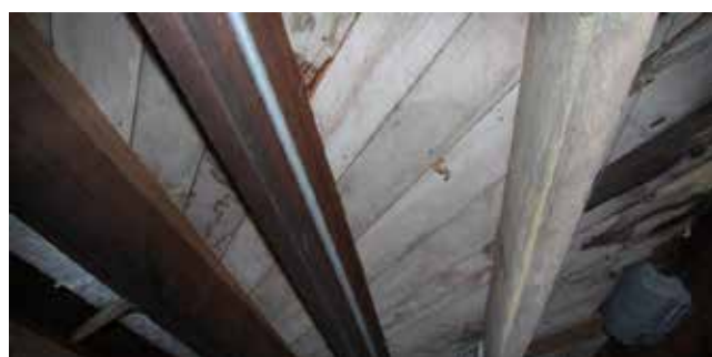
Figure 1.62 Diagonal floor boards of addition as seen from basement
