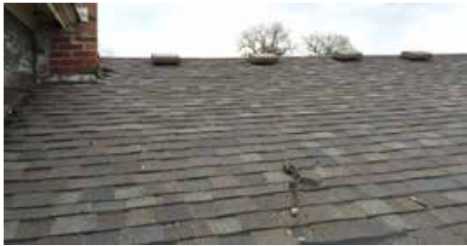
Figure 1.25 Image of roof over addition looking east.
