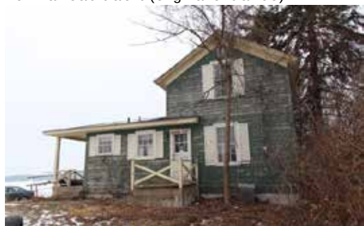
Figure 1.2 East façade showing addition and original house.
