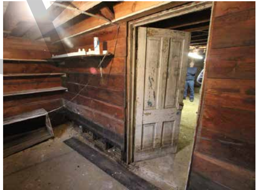
Figure 1.66 Original painted solid wood door in basement may have been relocated.
