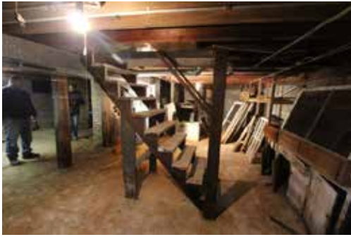
Figure 1.67 Stair at basement level
