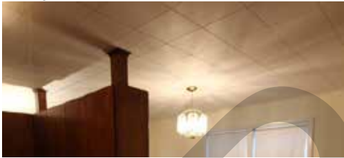
Figure 1.54 Acoustic ceiling tile in Kitchen
