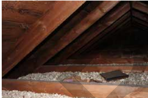
Figure 1.27 Attic of original structure with vermiculite insulation
