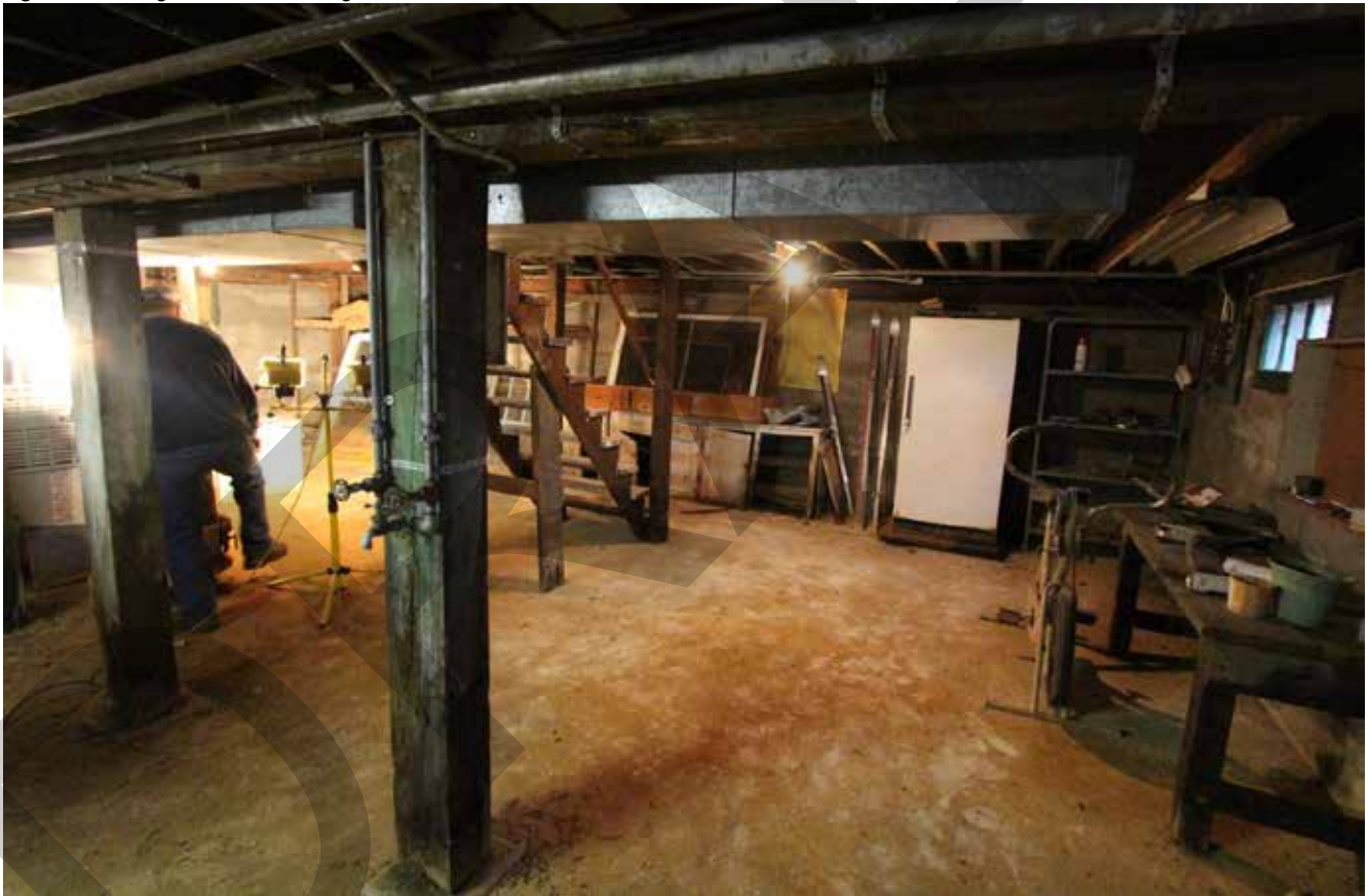
Figure 1.34 Wood columns and beam in center of Basement
