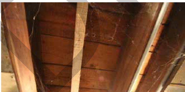
Figure 1.61 Horizontal floor boards of original building as seen from basement.
