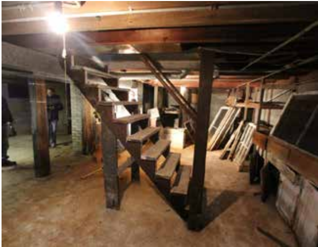
Figure 1.32 Left: Basement stairs below 1902 structure
