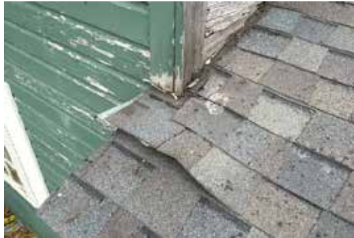
Figure 1.26 Roof intersects with original southern façade.
