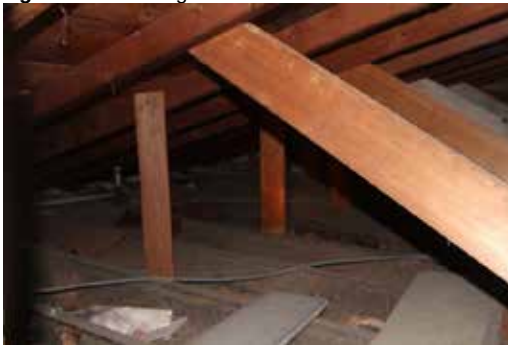
Figure 1.2 Attic above additions
