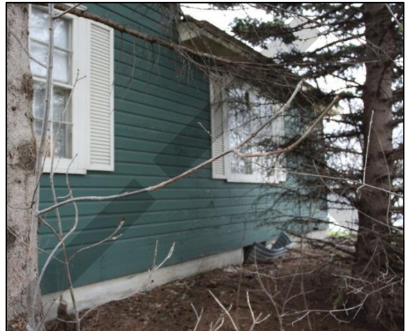
West side of original section (left) and addition (above).
