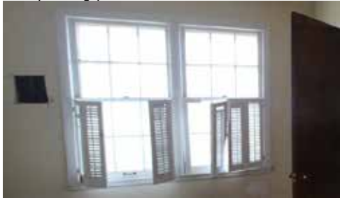
Figure 1.20 Window at south addition – bedroom
