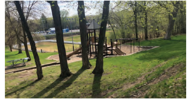
Existing playground outdated and inaccessible.
