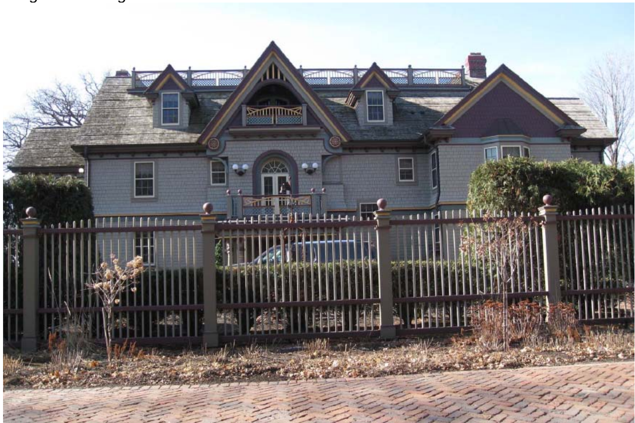
Image 1: Existing Residence at 532 Ferndale Rd W
