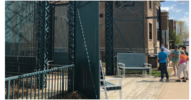
Existing entry gateway/sculpture.
