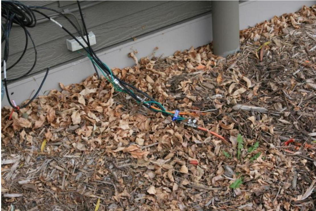
110 Grand Avenue S – Drops and ground wire partially exposed above ground near the building
