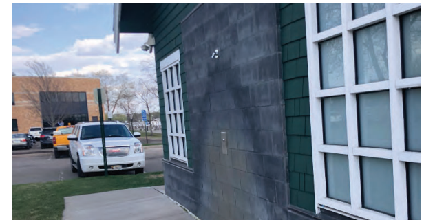
Existing showers hidden behind the building.
