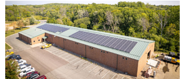
Public Works Facility
