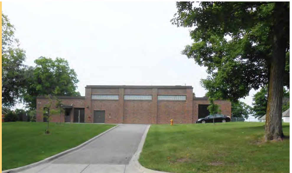
City of Wayzata WTP3
