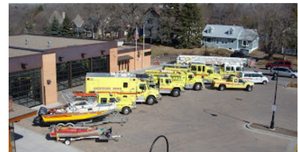
Fire Station & Associated Fleet
