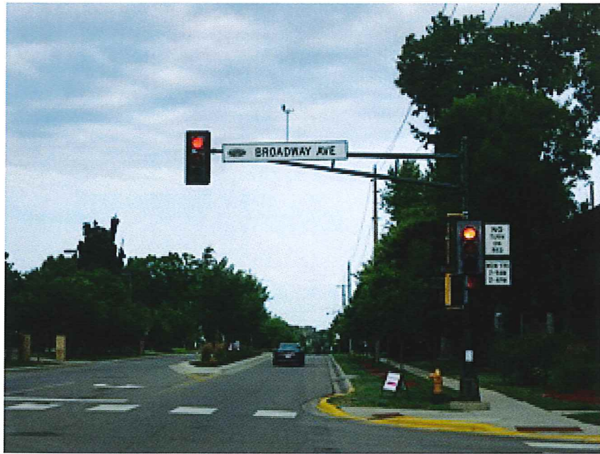
EXISTING/WAYZATA BLVD EASTBOUND @ BROADWAY AVE INTERSECTION
