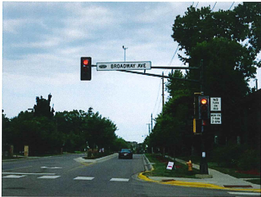
EXISTING/WAYZATA BLVD EASTBOUND @ BROADWAY AVE INTERSECTION
