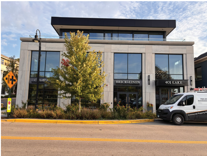
401 Lake Street Street Level (Existing)
