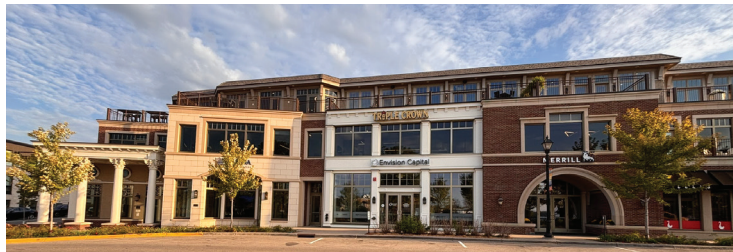
305 Lake Street Street Level | Commercial Use
