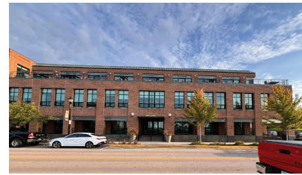
445 Lake Street Street Level | Commercial Use
