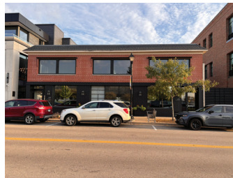
407 + 415 Lake Street Street Level | Commercial Use
