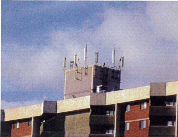
Antennas mounted on top of a mechanical room
