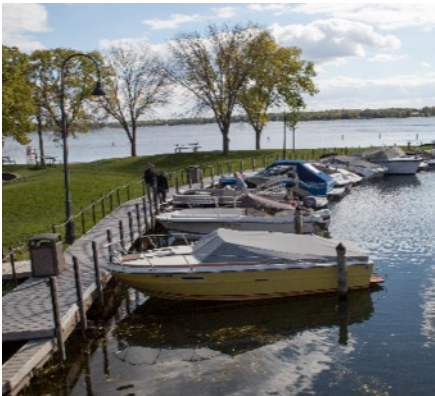
EXISTING BOAT SLIPS
