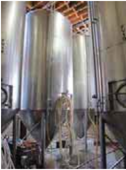
Stainless Steel Tanks for Fermentation
