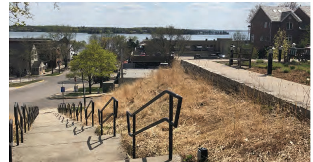
Existing Stairway leading to Lake Street
