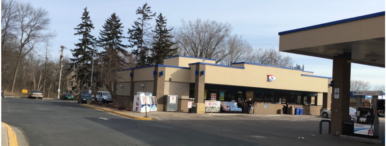
Photo Six West Side of Stationstore
