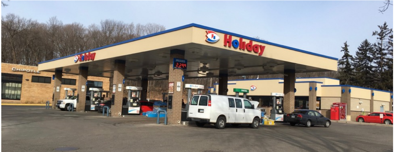
Photo Three Canopy and Stationstore from SE corner of the site
