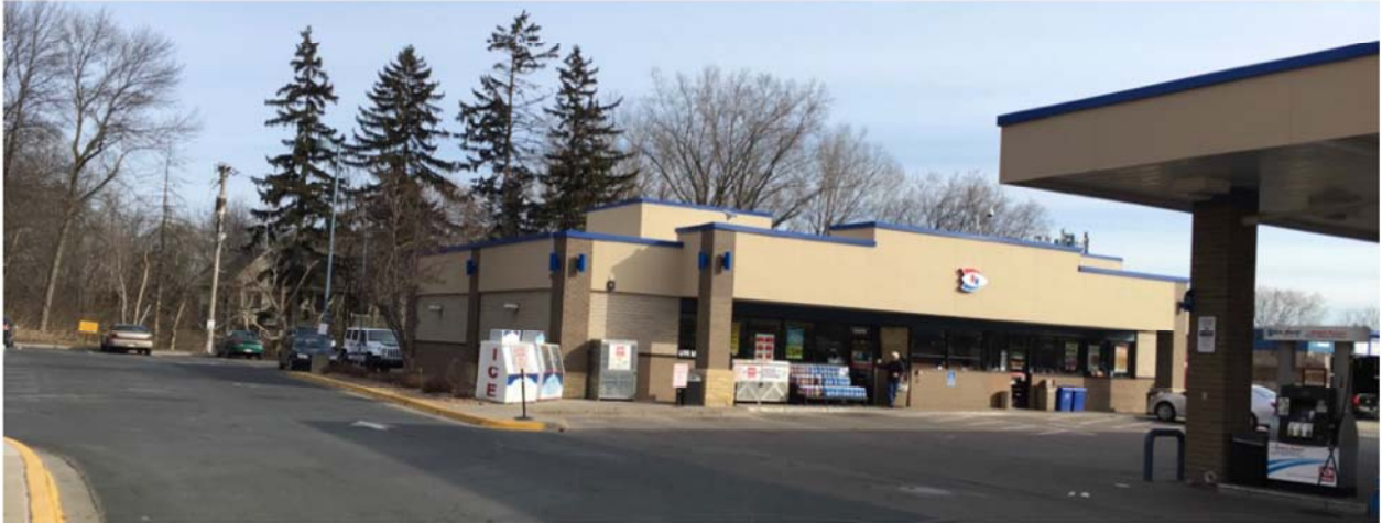
Photo Six West Side of Stationstore
