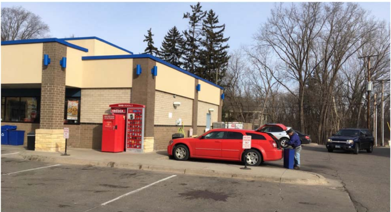
Photo Two East side of Stationstore
