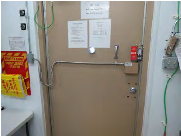
5 DOOR LOCK INSTALLATION PHOTOS SCALE: NONE
